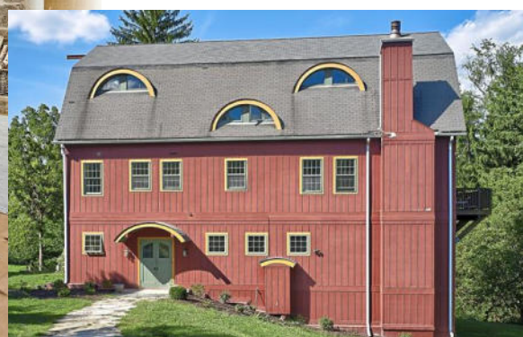
The lower level of the dairy barn still has stalls and a feeding trough.
